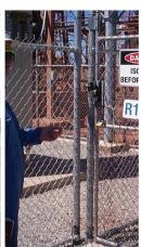
Concerns about magnetic radiation commonly require that working near air core reactors is restricted to locations where the magnetic field is less than 0.5 mT (depending on local regulations) and this is generally enforced by means of an HV cage fence or similar barrier.
